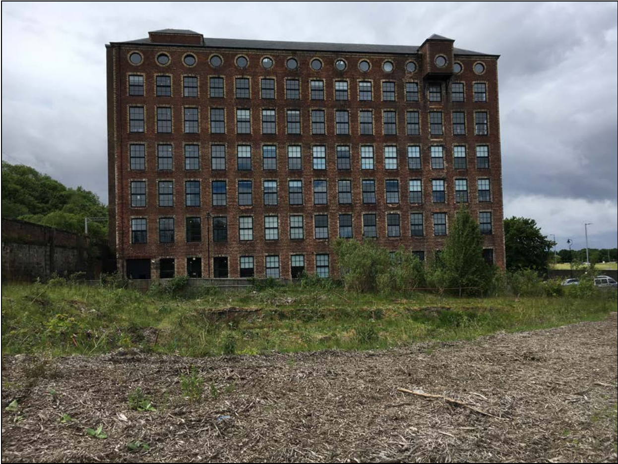
View of the 'A' listed Ropeworks building from within the site looking west across the site.
