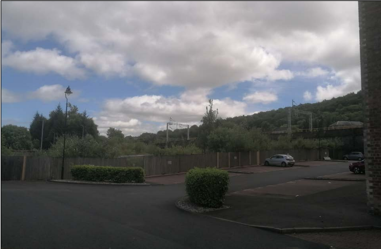
View of the site facing south-east from across the Ropeworks car park.
